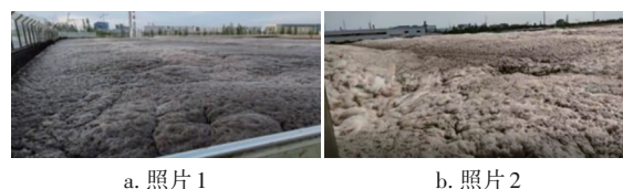
图3 某TCs生产废水生物处理系统出现泡沫剧烈现象 Fig.3 Foaming phenomenon in biological treatment system for TCs production wastewater
