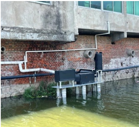
d. 岸边潜水式收集器实物 图 7 负压收集器大样及实物示意 Fig.7 Detail and physical schematics of negative-pressure collection units
